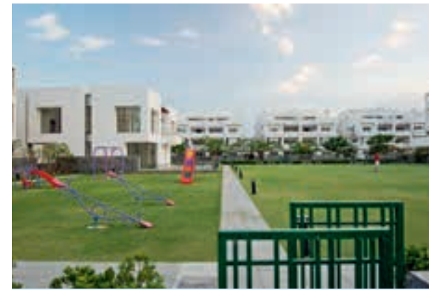
Four Clubs will provide recreational opportunity to the residents. One is already operational while two are under construction
